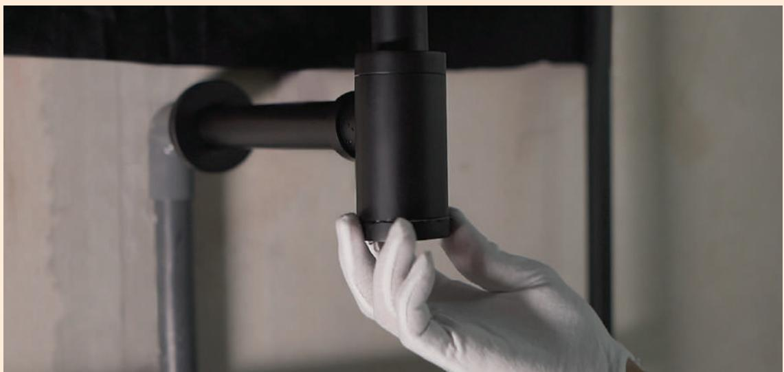
To drain the P-trap open the bottom cap by twisting it anti-clockwise. Prepare a container to hold the trapped water inside of it.
